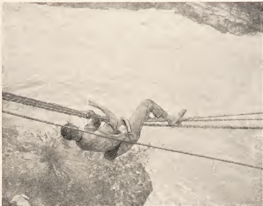
NATIVE CROSSING ROPE BRIDGE
